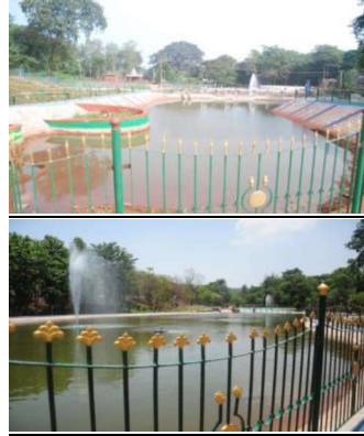
RWH structure for ground water augmentation in the area
