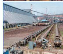
Base mix plant
