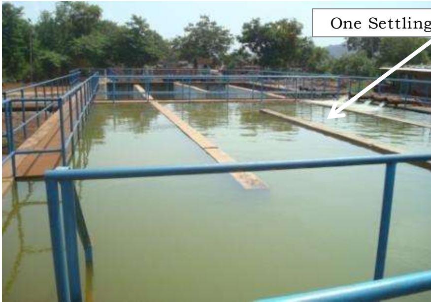
One Standby Settling Tank
