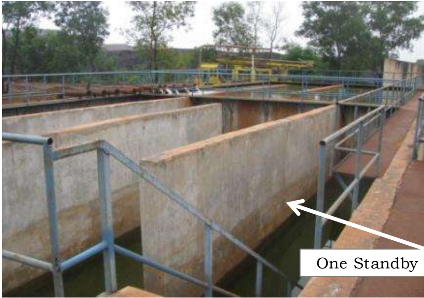
One Settling Tank in use
