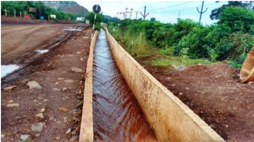
Garland drain concrete culvert
