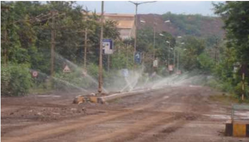
Photograph showing Dust suppression using Stationary as well as Mobile water sprinklers
