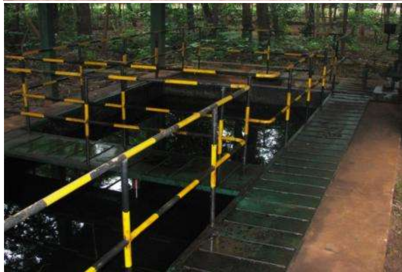
Oil and grease Separation pit
