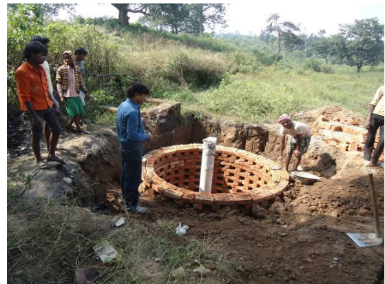
Artificial ground water recharge pit (Bore well) in Birlor village
