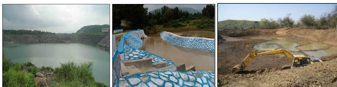
Rainwater harvesting structures
