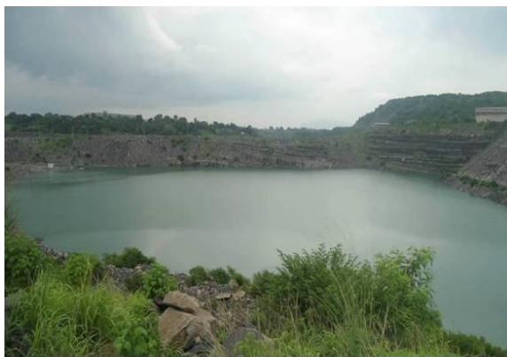
Abandoned mine pit as RWH pond
