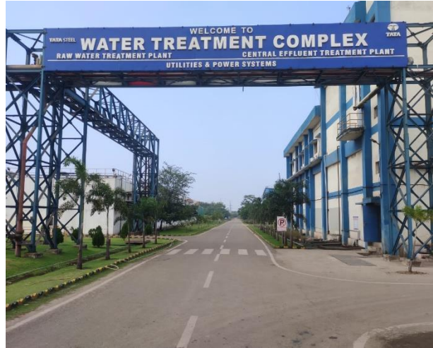
Water Treatment Complex (RWTP and CETP)
