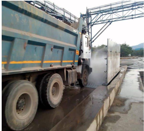
Wheel Washing facility at MRP
