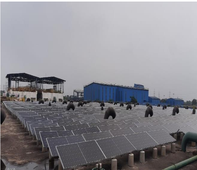
PV Solar module installation at RWTP Roof top
