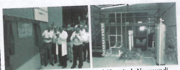
10 KLD ETP at TATA Steel Hospital, Noamundi
