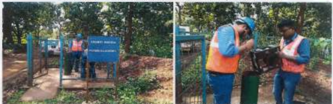
Piezometric borewell installed at Katamati entrance gate, Katamati Mine
