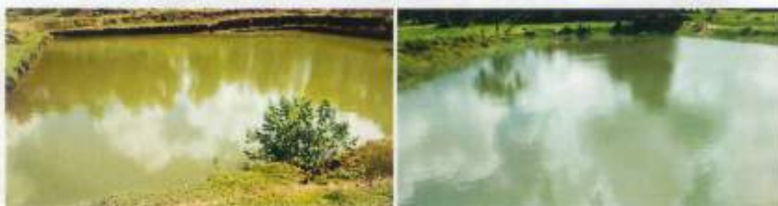
Water harvesting Pond at Kolahundala & Narayanpur village, Katamati Area
